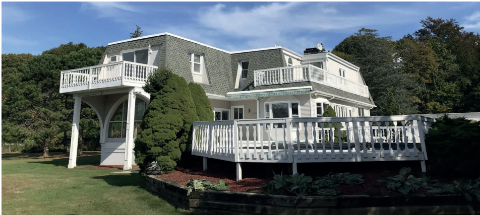
Center Moriches—$799,900 Spacious 4 bedroom, waterfront home on Areskonk Creek. 200 ft. bulkhead with dock and boat lift.
